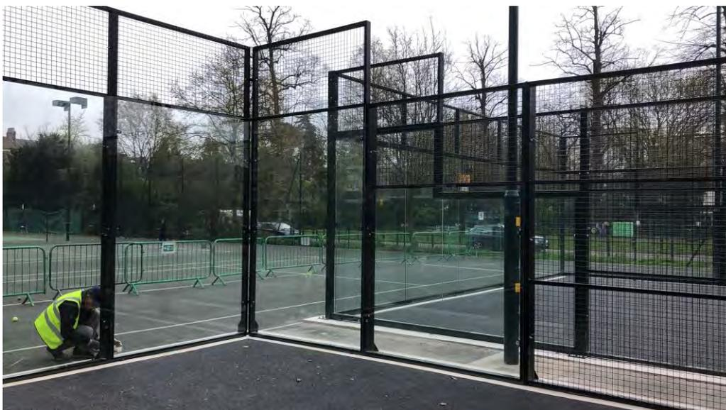
Glass and weld mesh panels are supported by steel posts or framed steel panels with base plates for fixing to the concrete ring beam.
