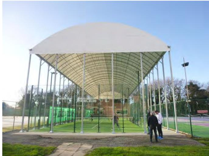
A range of structures are available which comprise steel portal frames sitting outside the fence / rebound wall elevations of the padel enclosure with single or double skin membrane with or without full or partial drop down walls.
